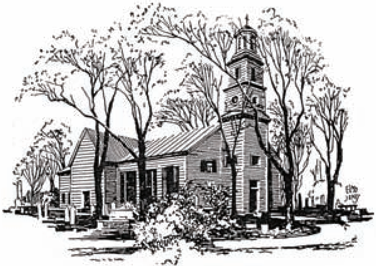
St. John's Church Erected 1741
